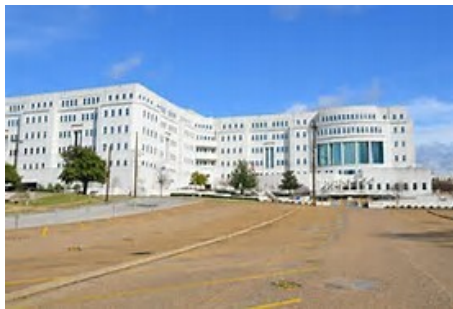
Gordon Persons Education HQ Bldg.
